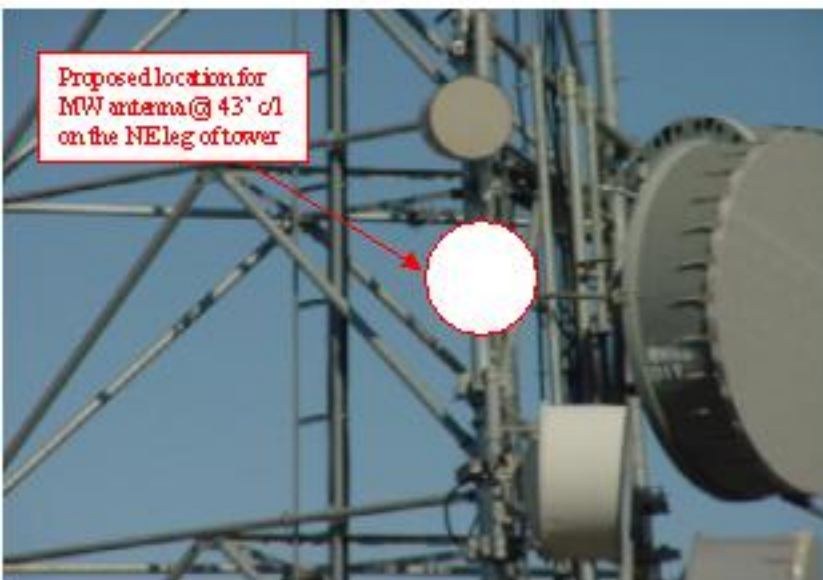
Close up view of Elsinore Peak tower and proposed location for MW antenna.
