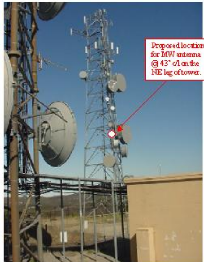
View of entire tower at Elsinore Peak and proposed location for MW antenna
